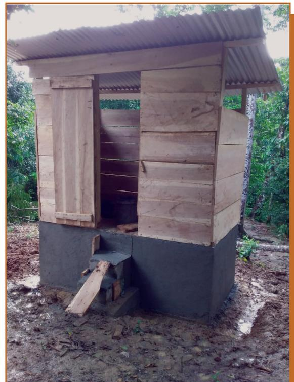
cement- block base built off the ground. Inside, are two adjacent holes where a cement-molded seat stands over one of them. The system separates the urine from the dry matter, converting excrement into fertilizer after about 4 months. It serves a dual purpose.
